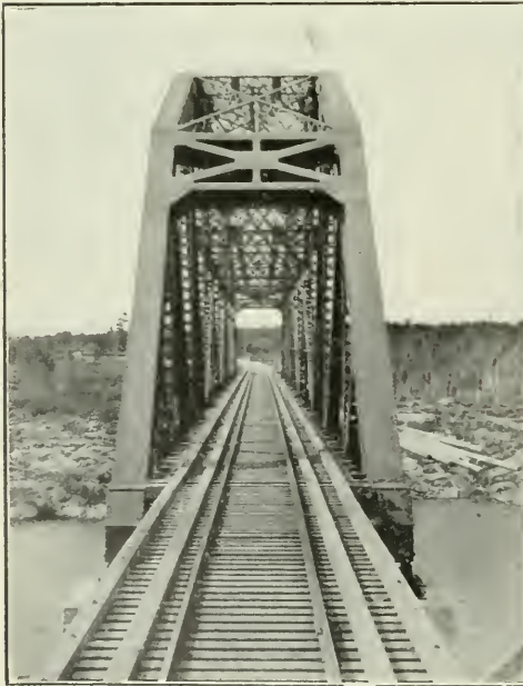
THE BRIDGE OVER THE PICKEREL RIVER
